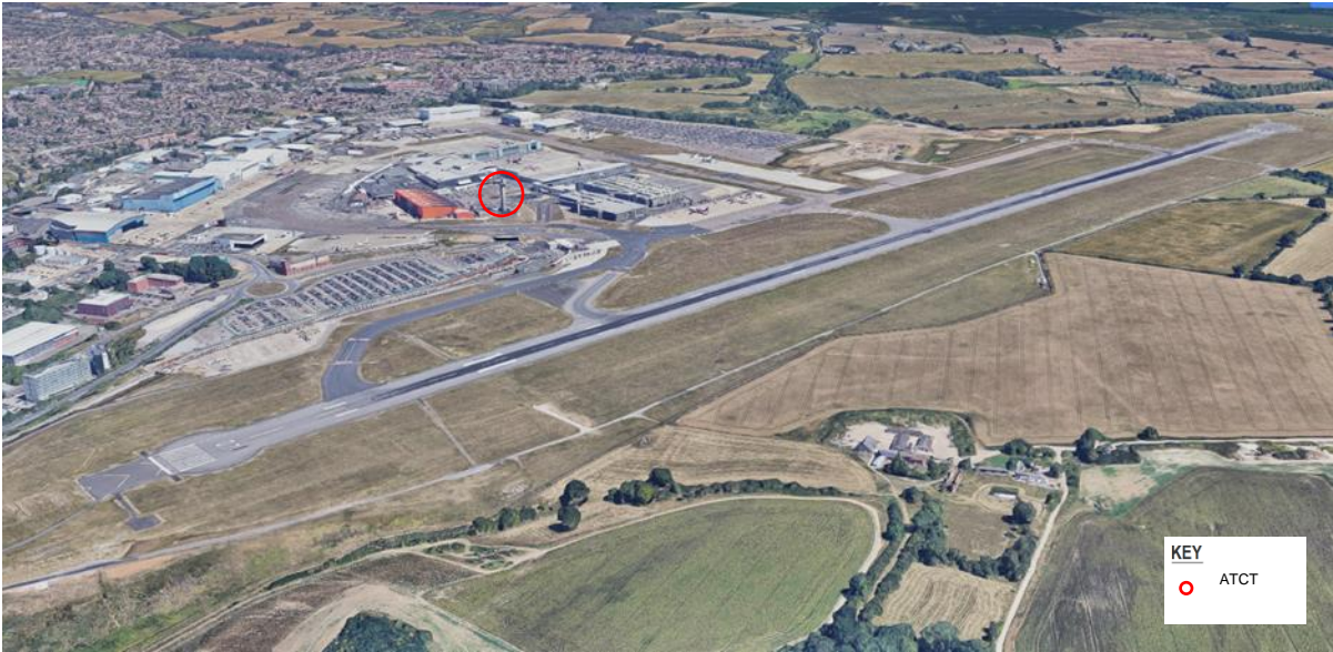
Figure 4-2 Existing Site Context Aerial Photograph (Source: www.google.com/maps)
